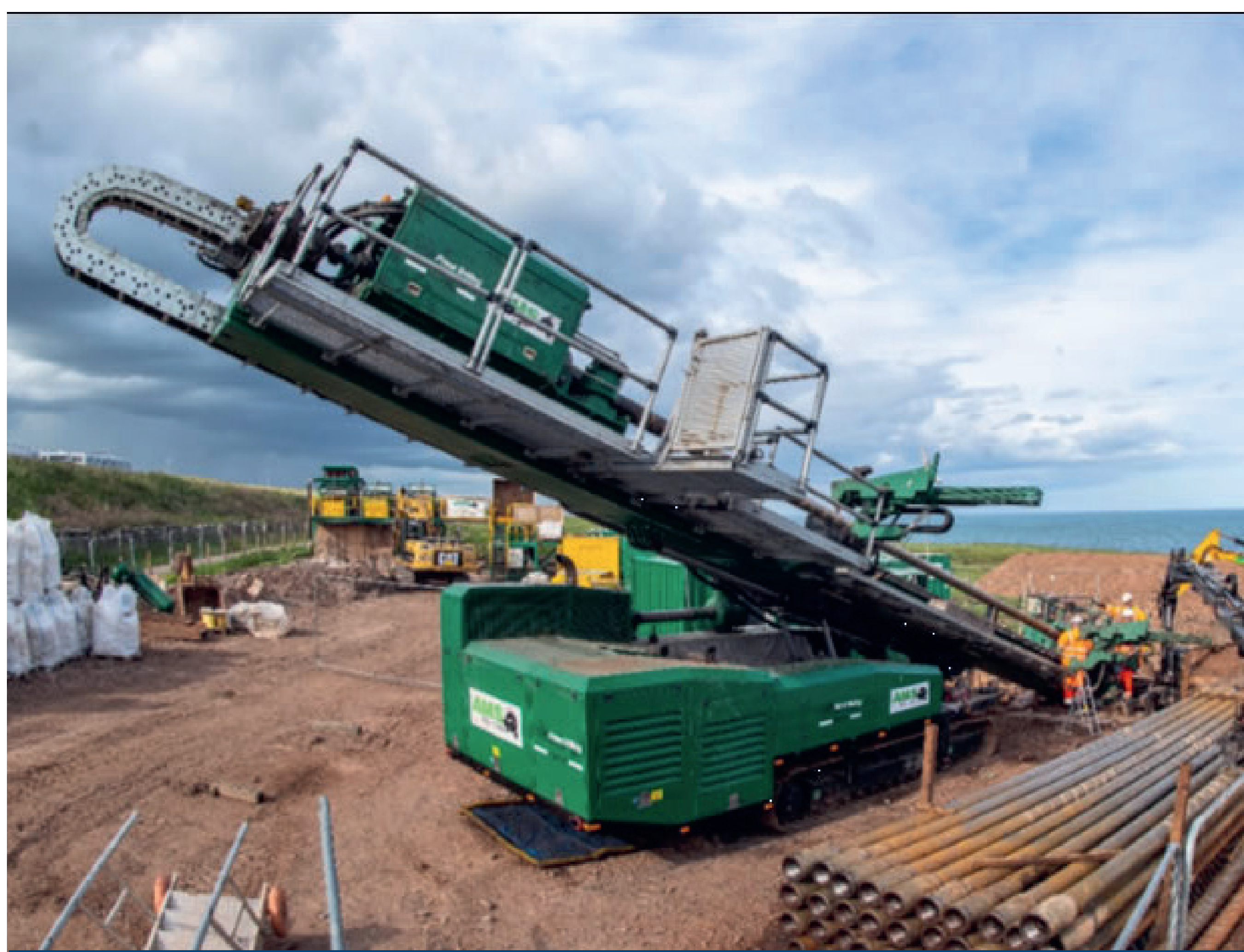
Horizontal Directional Drilling Rig (image: AMS Trenchless)
