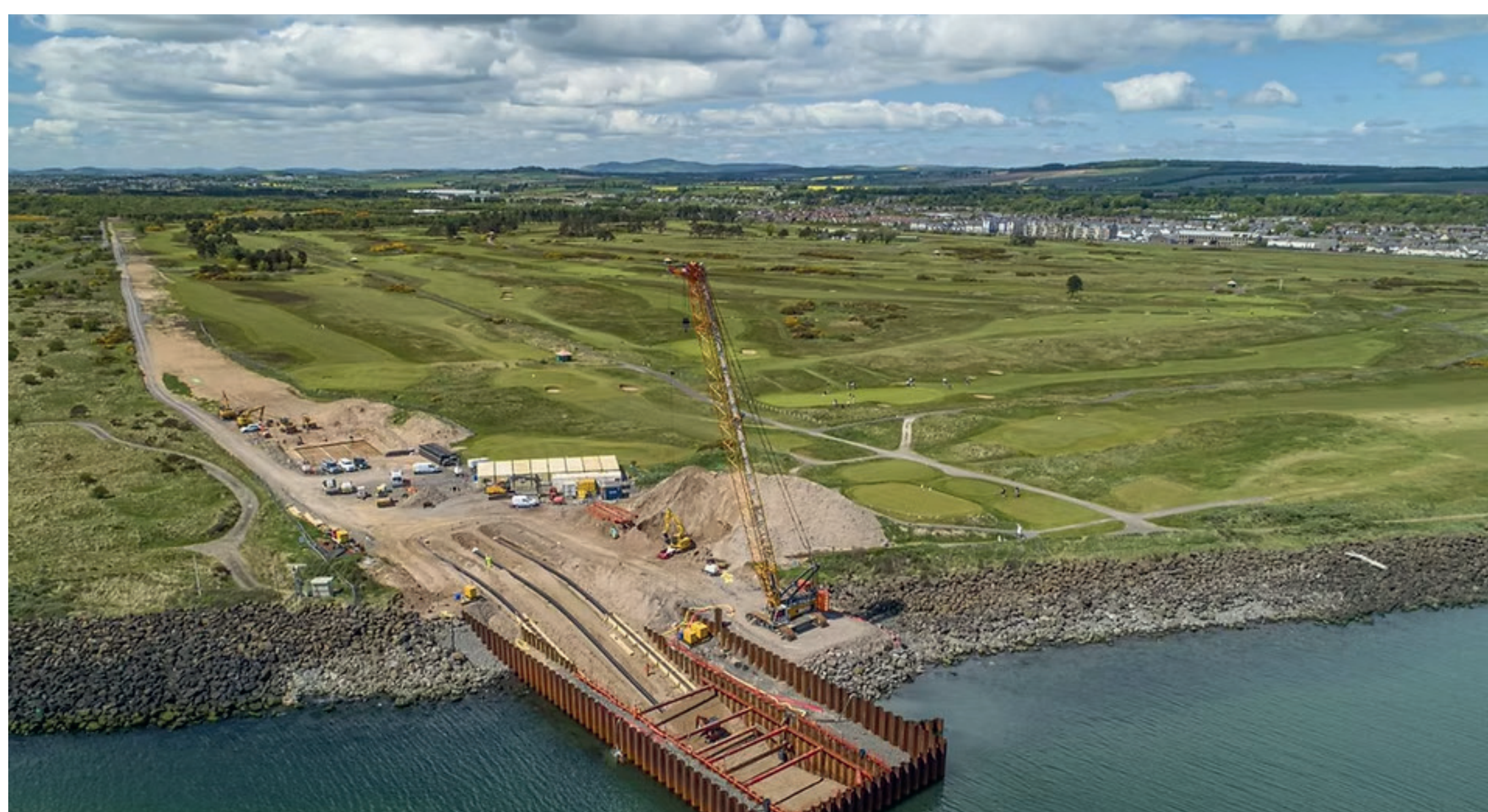
Example of open trench technique during installation
