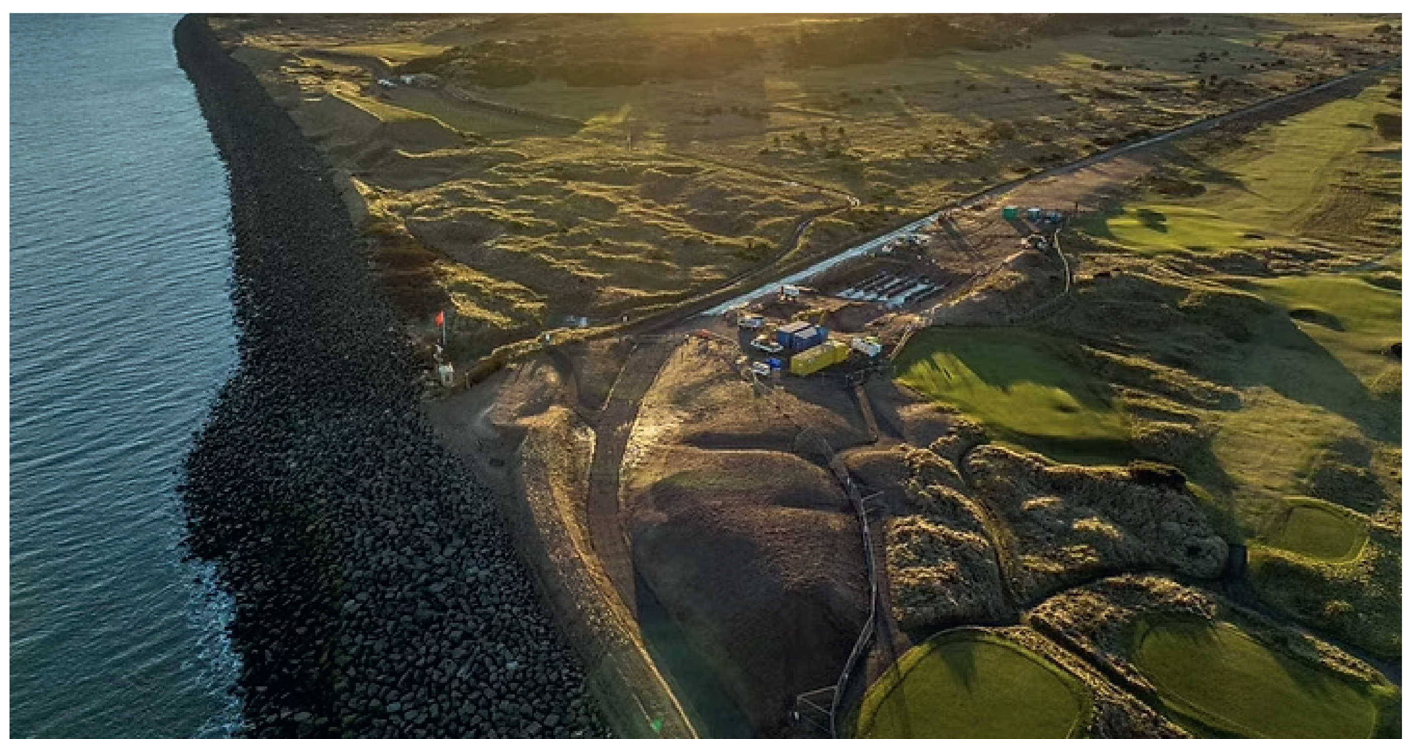
Same example post installation
