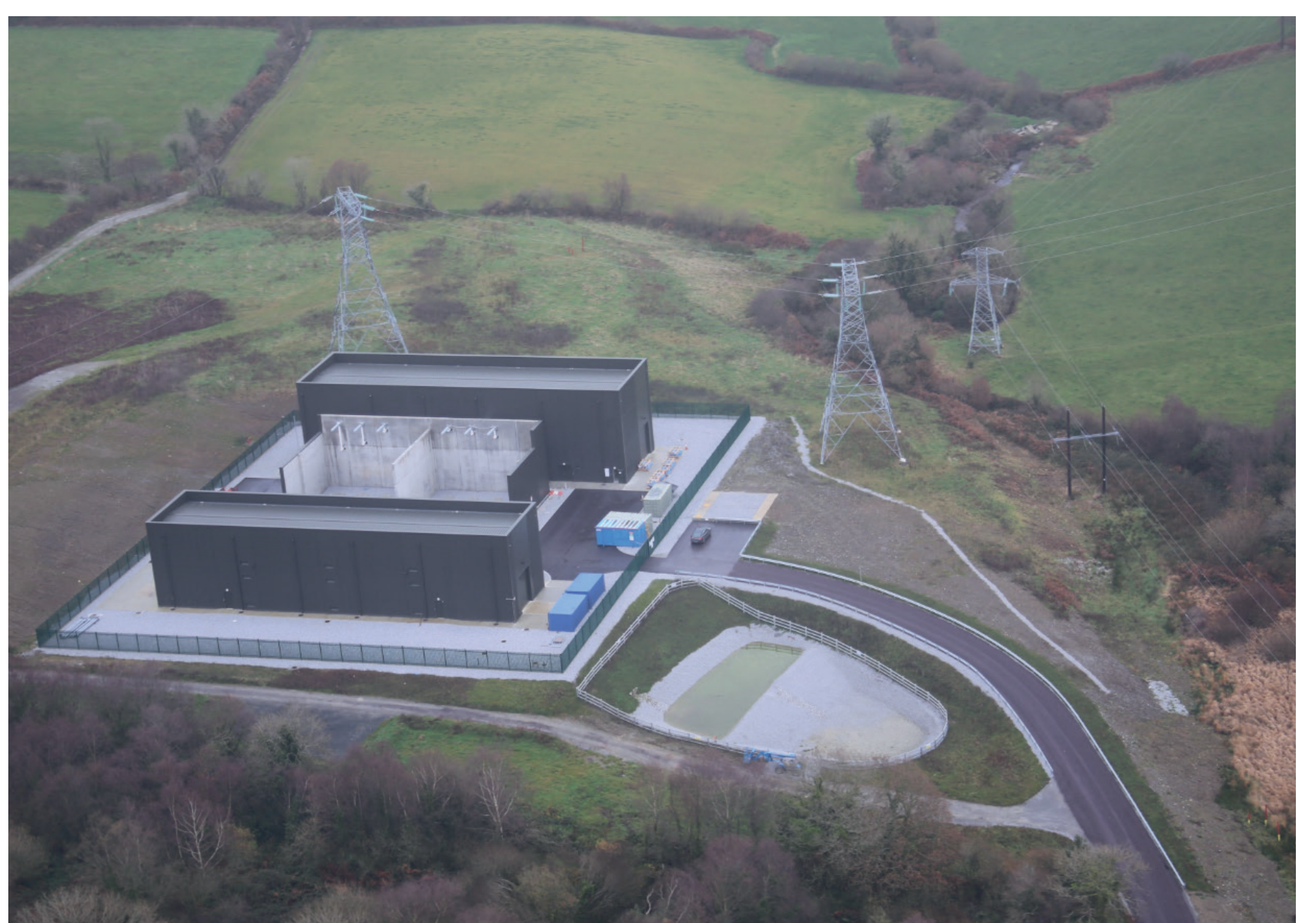
Substation with Gas Insulated Switchgear
